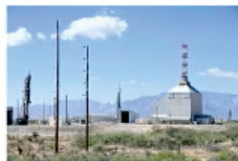
WSMR LC-36 with launch rails and towers
