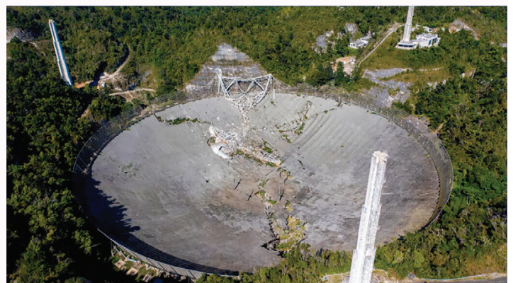
Arecibo after collapse
