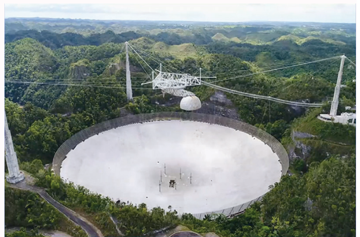
Arecibo before collapse
